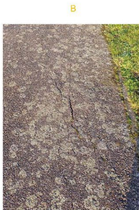
East side pathway on entrance to Summerfield Drive Cracking of pathway
