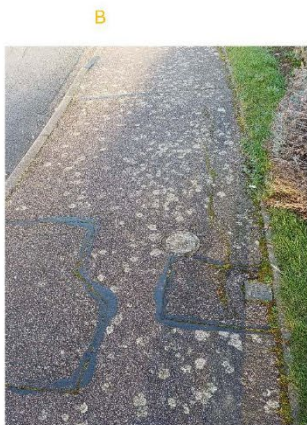
East side pathway on entrance to Summerfield Drive Cracking of pathway
