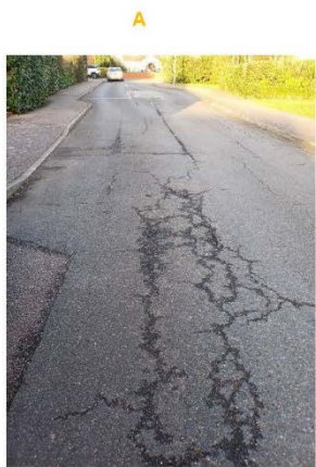
Entrance to Summerfield Road Cracking in road surface
