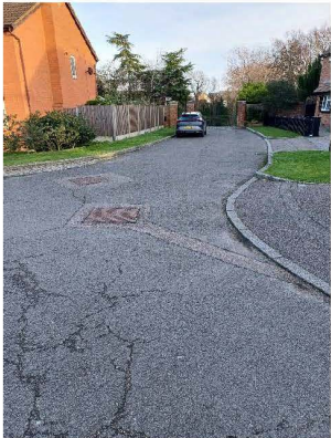
Bellamy Road Cracking in road surface No tarmacked pathway on either side therefore pedestrians use roadway due to state of grass area which also cannot be used by wheelchair users or those with wheeled buggies.
