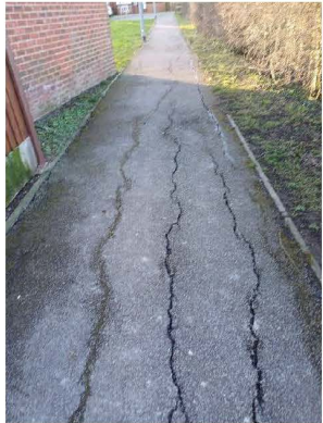
Pathway between Summerfield Road and Hillcroft Severe cracking of surface
