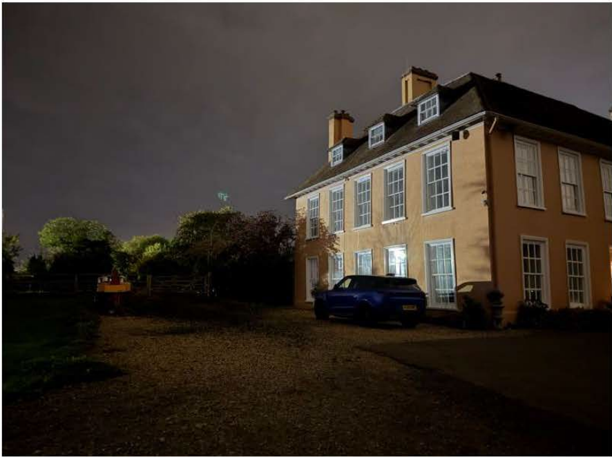
Images of the bright flood lights at night from Wootton House directly illuminating the facade
