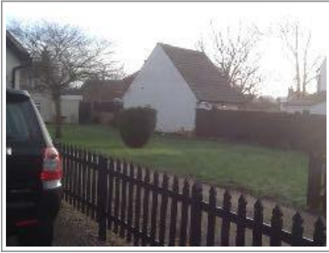
The back of 1A Potters Cross looking onto proposed site( from 78 Bedford Road)
