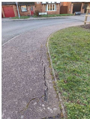
Summerfield Road footpath south of Barnes Road Cracking of pathway
