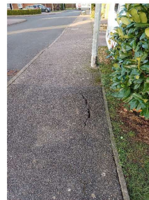
Summerfield Road footpath south of Barnes Road Cracking of pathway
