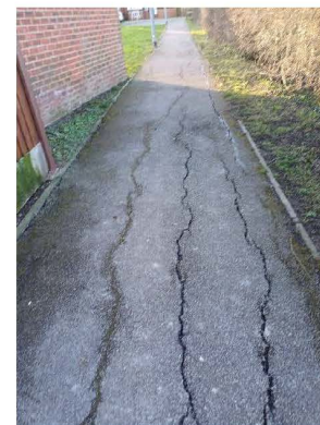
Pathway between Summerfield Road and Hillcroft Severe cracking of surface
