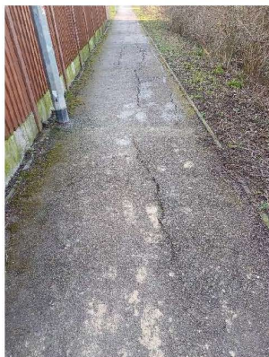
Pathway between Summerfield Road and Hillcroft Severe cracking of surface
