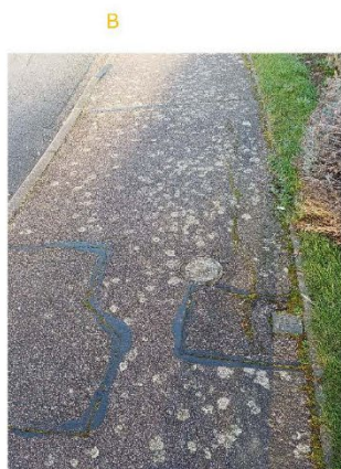
East side pathway on entrance to Summerfield Drive Cracking of pathway
