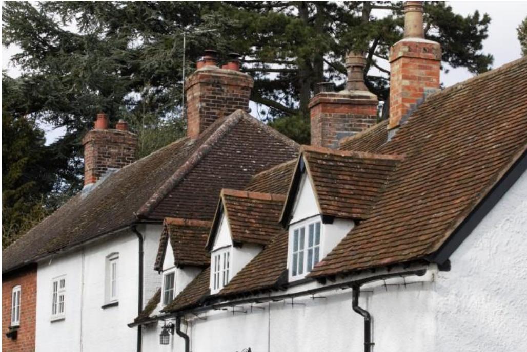
Plate 63 The dwellings in the foreground illustrate the use of clay roof tile, with clay ridges and valley tiles.
