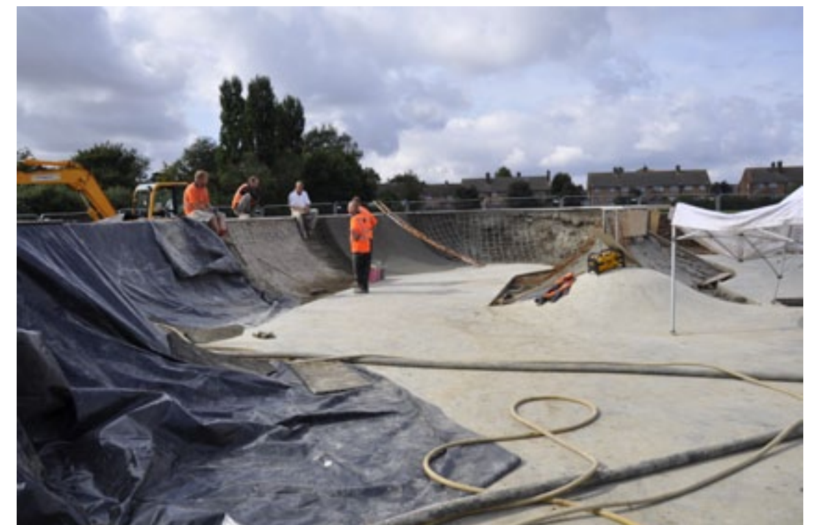
Just waiting for another load of concrete to be delivered
