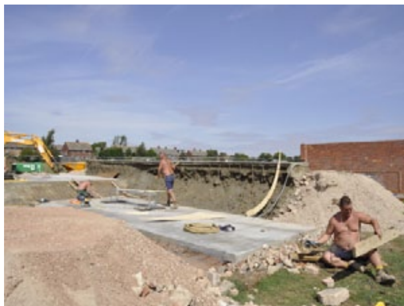
Frames being prepared for cement to be sprayed along the length of the ramp
