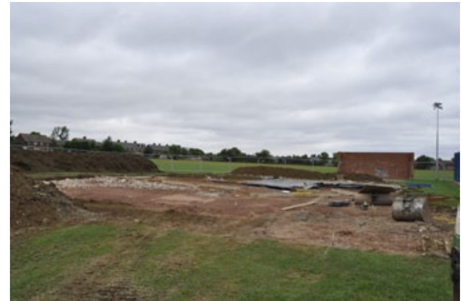
End of week 1, concrete left to dry out
