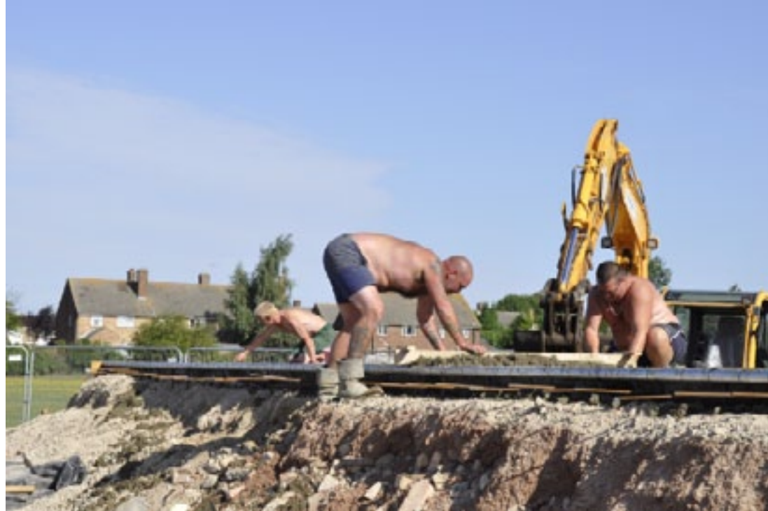
Cement being laid and smoothed off on top of ramp
