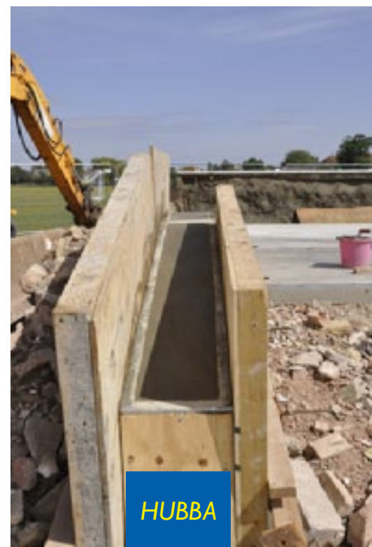
Frames being prepared for cement to be sprayed along the length of the ramp
