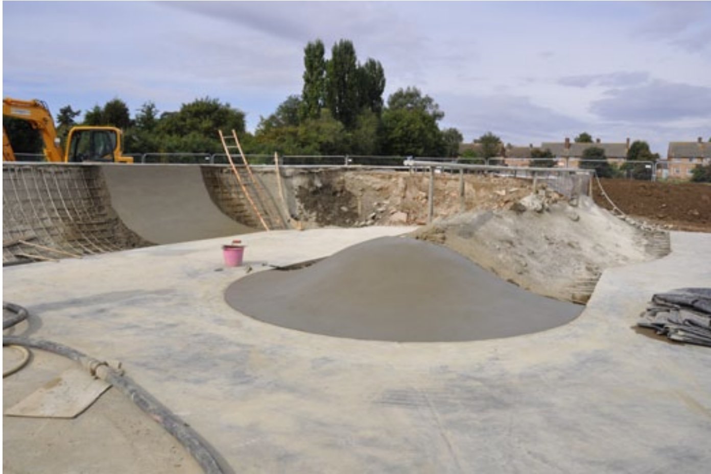
End section of bowl and one section of the end ramp completed
