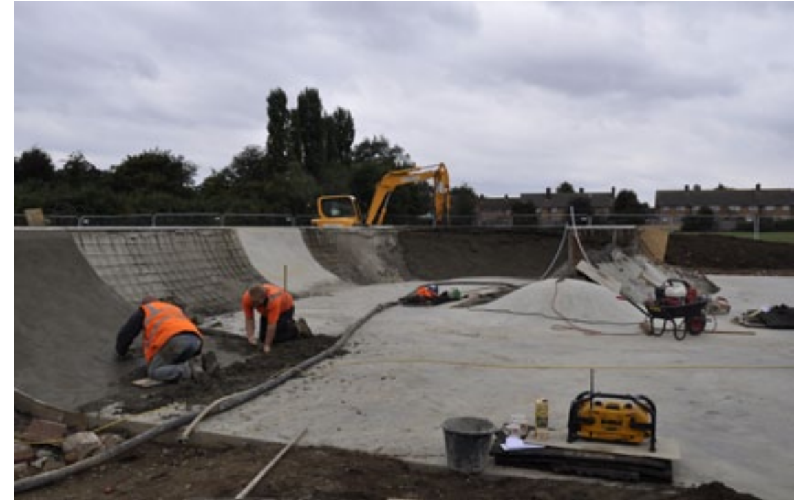
Another section of the end ramp leading into the bowl being completed
